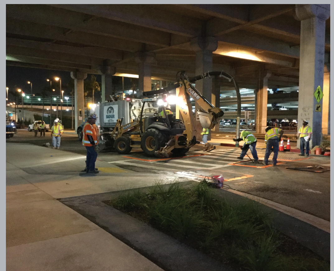
Our Underground Division crews managing pothole operation in the Central Terminal Area.
