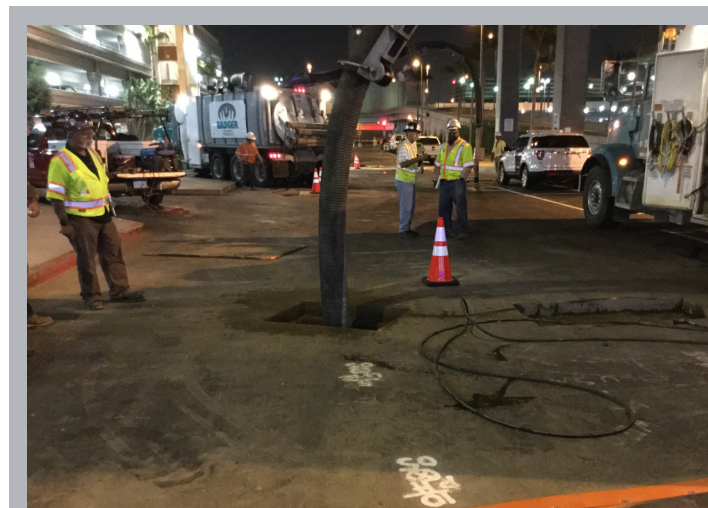
Utility information was obtained by using vacuum trucks to avoid utility strikes.
