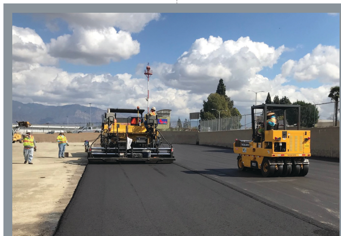
Paving at San Gabriel Valley Airport
