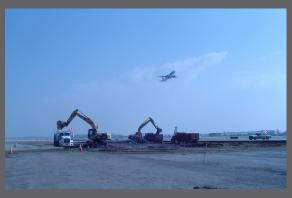
Griffith Company began work on this \$9 million contract in early 2001. As part of the project, our crews widened a two-lane road into a six-lane road with a median. Completing this work required the demolition of all toll booths, construction of a post-tension box, reservoir and pump-station facilities. This in turn required the installation of 5,000 linear feet of storm drain and 4,500 linear
