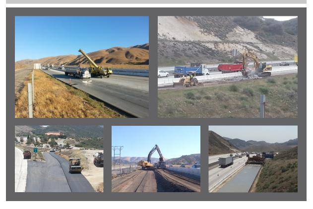
Griffith Company and its joint venture partner, Coffman Specialties, constructed this resurfacing and restoration project with the primary goal of extending the service life of the pavement structure. The project consisted of pavement rehabilitation for 16 miles in the northbound and southbound directions from south of Vista Del Lago Road to the Kern County Line near the Town of Lebec, CA.
