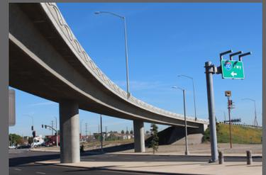
This project combined two closely spaced intersections into one and constructed a new bridge flyover off-ramp from the northbound I-110 freeway onto Harry Bridges Boulevard. The structure is a 465-foot-long four-span cast-in-place concrete box girder bridge. The jobsite is located within C Street ramps of the I-110 freeway and the intersection of John S. Gibson Boulevard, Harry Bridges
