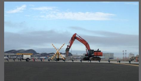
The project was a key runway reconstruction and Runway Safety Area improvement project for LAVA which included the removal and replacement of Runway 6L-24R and Taxiway AA, a new pre-cast box culvert, reconstruction of the North Access Road, FAA Access Road and AOA fence improvements. The 240 day schedule was constructed in six different phases including a 55 hour shutdown of two of the four runways at LAX to construct a portion of the Runway 6L-24R that incurred on 6R-24L. In another
