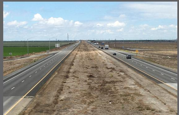
The Wheeler Ridge Project was a 45-day contract to lay 60 lane miles of Rubberized Hot Mix Asphalt (RHMA) paving. To meet this aggressive milestone, a well-choreographed pre-bid schedule was put together utilizing two traffic control crews, with contract work taking place
