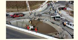
Levi Pivovoroff Bakersfield Roundabout: "Placing Concrete for the JPCP Roundabout Utilizing a 32M Pump".
