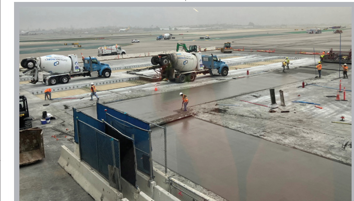
P-501 Concrete Placement at Alaska Terminal 6 Apron Paving in LAX Airport
