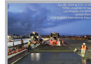
Lean Concrete Base Placement on MSC South in LAX Airport
